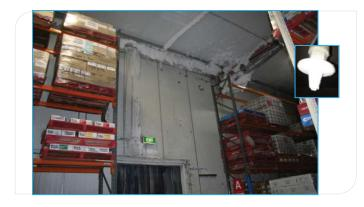
It is generally accepted that ASD is the best (only) solution for refrigerated storage facilities. However, there are some typical problems associated with applying ASD in these applications. Over time, ASD sampling points and pipe within the sub-zero area can become blocked causing air flow issues and inoperative detection of smoke. In some instances the only solution is to remove the iced up section of the ASD pipe network and fit a new pipe.
